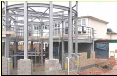
Café area - Steel frame in place. Brickwork and Blockwork underway.
