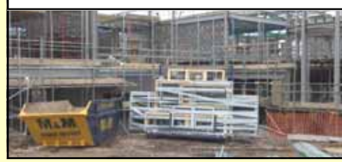
Front Elevation - Brickwork and Blockwork underway - external windows delivered
