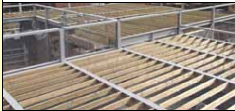
Roof timbers in place and ready for weather proof coverings
